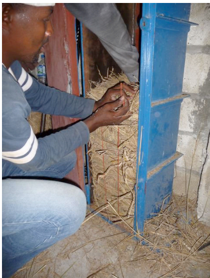
Straw bale being tied off in a steel compression mould.
