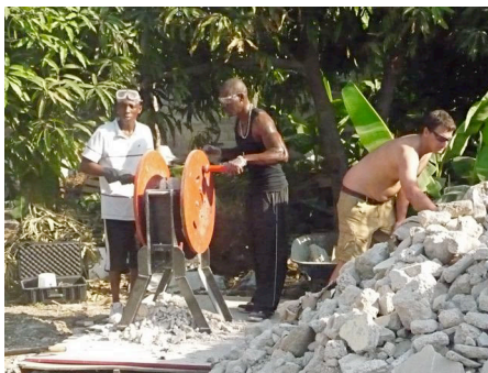
Crushing rubble into usable aggregate
