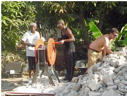
Crushing rubble into usable aggregate
