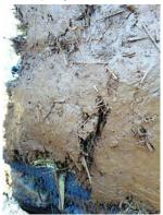
opposed to it steel mesh counterpart. The straw reinforced clay plaster (1.5" chopped straw) applied could not sufficiently penetrate the steel mesh size and resulted in plaster "buckling" This was also a pronounced condition with the 1" diamond mesh used on the TiKay strawbale building in Haiti.
